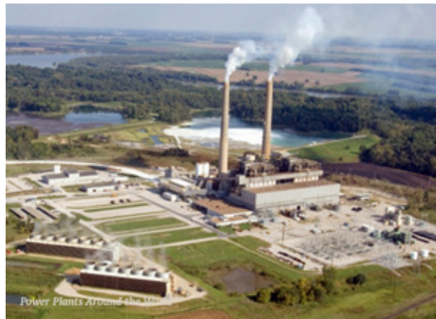
Figure 4 - AB Brown Power Plant, Indiana
